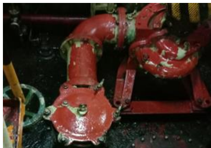
Gambar Pompa Ballast
